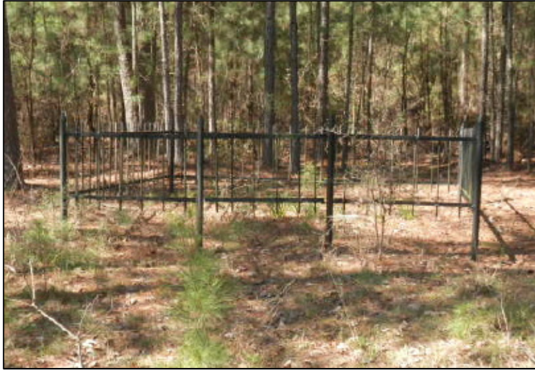
New fence installed around the Wallace graves
